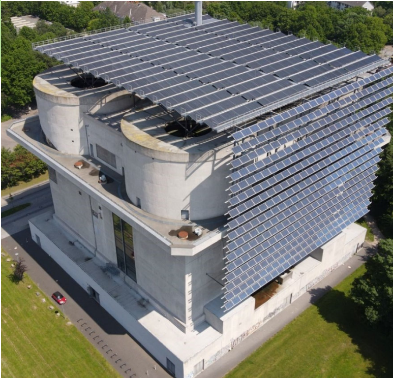
For roof systems, the statics and load-bearing capacity of the building play a decisive role. Photo: AboveSurveying_Energiebunker/HamburgEnergie
