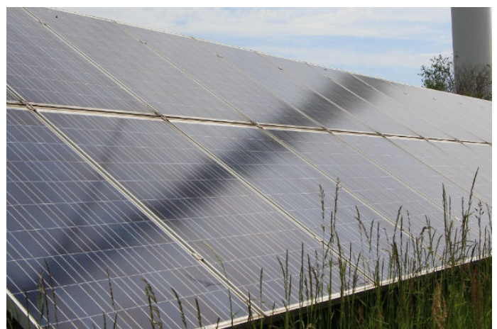
Shading by a nearby wind turbine
